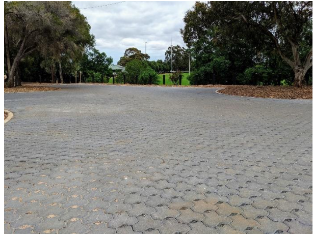
Figure 15: Permeable pavers at Bell Yett Reserve car park, City of Burnside
