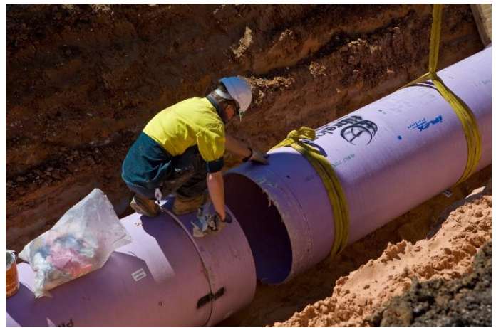
Figure 3: Glenelg-Adelaide Pipeline installation (GAP) (credit: Mark Dohring).
