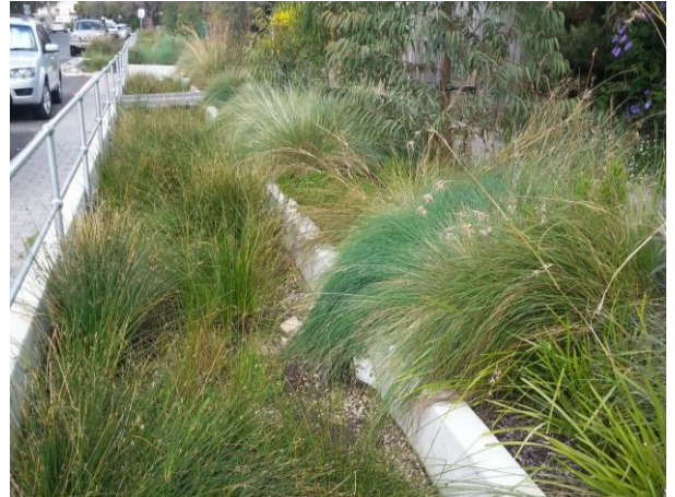
Figure 8: Raingarden, Randolph Ave, Fullarton City of Unley (credit: Water Sensitive SA).
