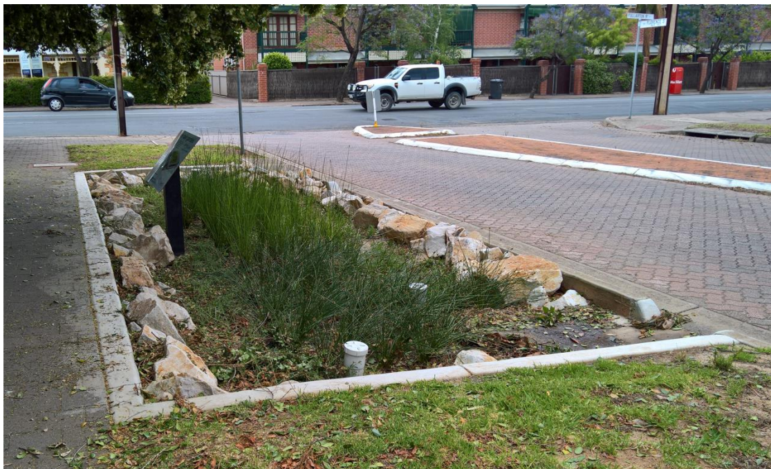
Figure 1: Raingarden, Florence Street, Fullarton, City of Unley. One of three raingardens in this location that provide additional green space and have indigenous plants to attract wildlife. These raingardens reduce local flooding and improve water quality going into Parklands Creek. (credit: Environmental Protection Authority South Australia).
