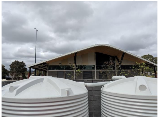
Figure 10: Rainwater tanks, Glenunga Hub, City of Burnside.
