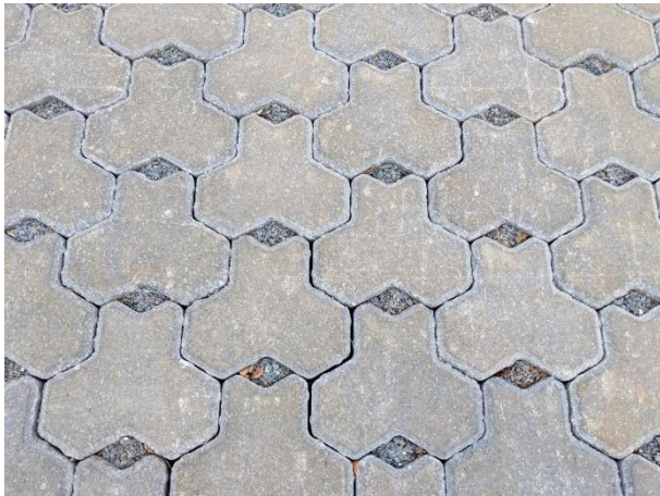
Figure 9: Permeable paving, Tregenza Oval, City of Burnside.
