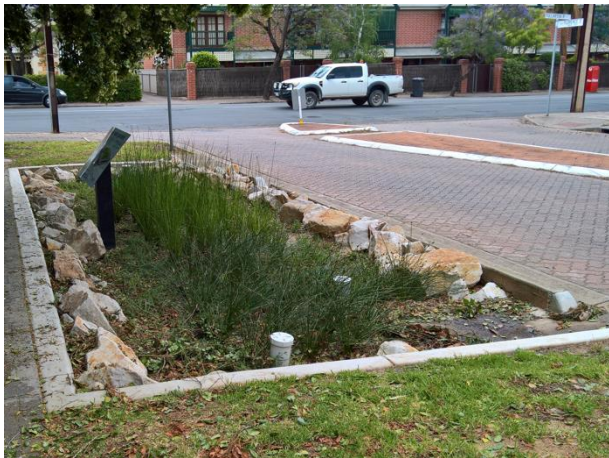
Figure 16: Raingardens & bioretention filters, Florence St, City of Unley (credit: Environmental Protection Authority South Australia).
