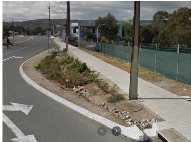
Figure 17: Raingarden installation, Smart Road, City of Tea Tree Gully
