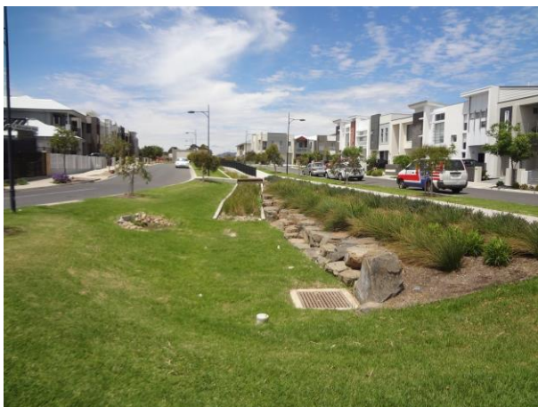
Figure 11: Detention basin (credit: Water Sensitive SA).
