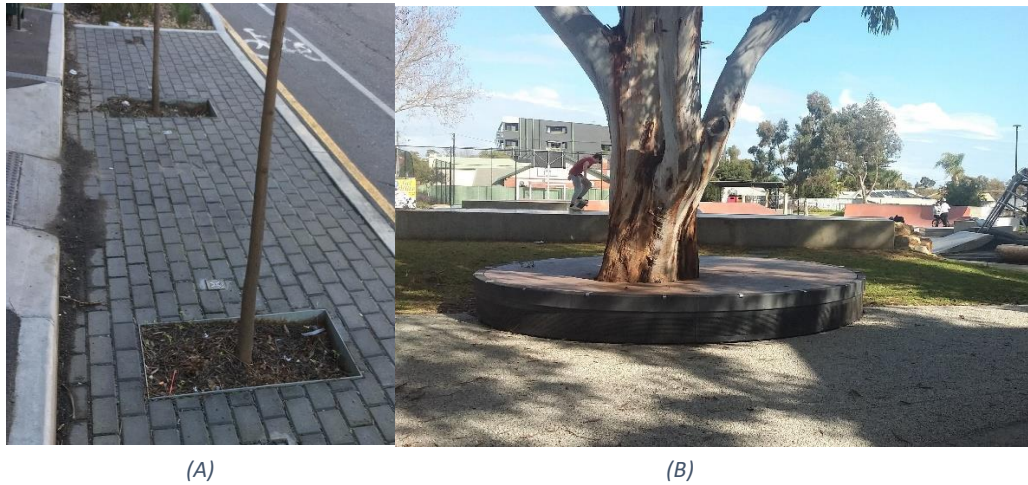
Figure 8: An example of (A) permeable paving, where the water seeps directly into the tree root zone below, and (B) porous paving, which is porous aggregate and has a similar function. Here it surrounds and protects a significant gum tree in Prospect.
