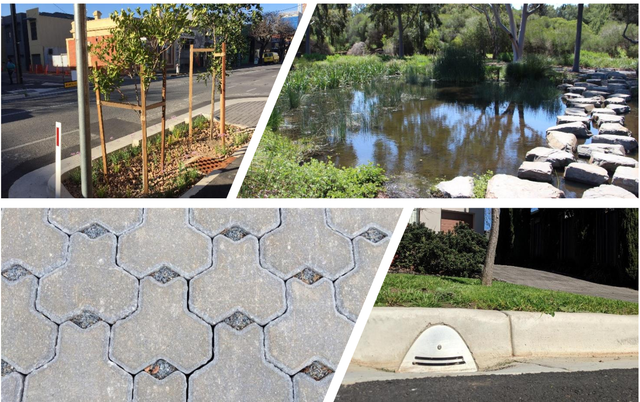
Examples of WSUD in Resilient East – a bioretention system, wetland, permeable paving and a Treenet inlet
