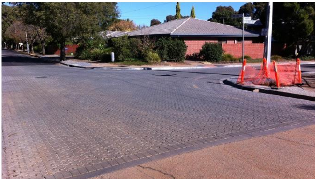
Figure 7: Example of permeable paving at Mitcham Council, South Australia. Image taken from (Lawry et al. 2017)
