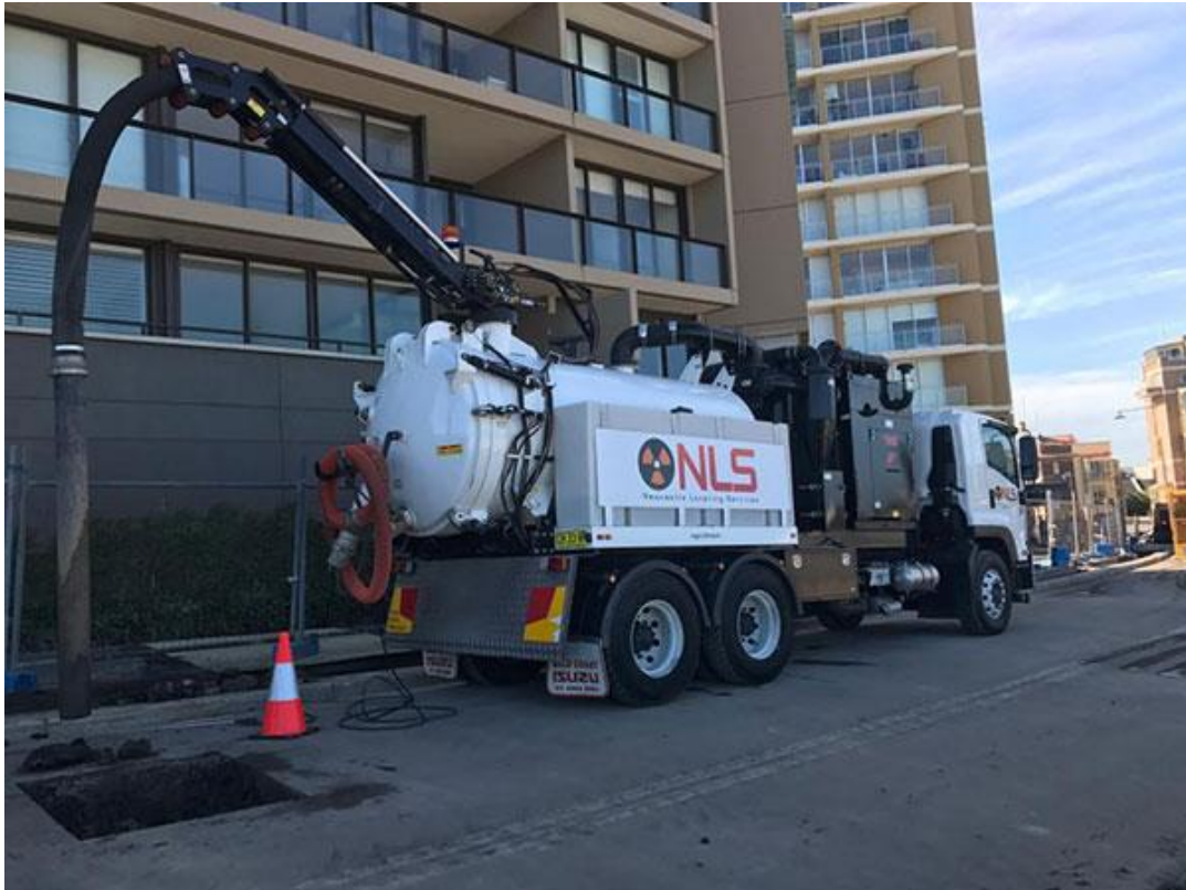
Figure 15: Vacuum excavation to expose utility services in the city. Image: https://www.newcastlelocatingservices.com.au/vacuum-excavator-hire
