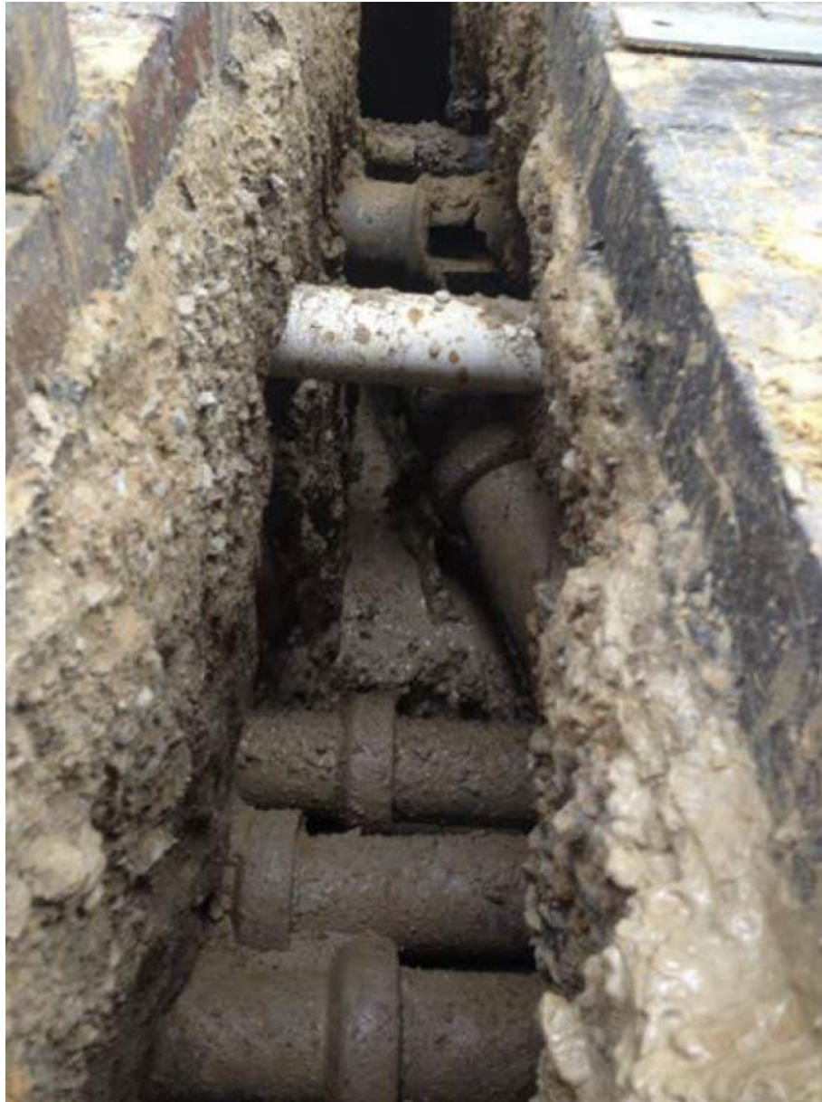
Figure 12: Example 1 of the extent of services in a city underground space, Bank Street Adelaide.
