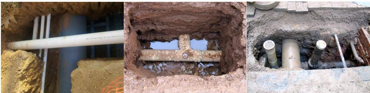
Figure 16: Utilities exposed by vacuum excavation. Images: http://www.statewidehydrojet.com.au/sa/shj/main/hydro-excavation-adelaide/
